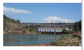
PDR's hydropower potential, but it has also striven to achieve flood protection, implement lift irrigation, facilitate lake fishery, and develop Lao PDR's tourism industry. The Nam Ngum Dam has a capacity of 155MW and generates most of Laos' electricity, including all the power used in the capital, Vientiane. The reservoir surface area at H.W.L is 370 km2 with Gross Storage Capacity of 7.03Billion m3 and Effective Storage Capacity of 4.7 Billion m3
